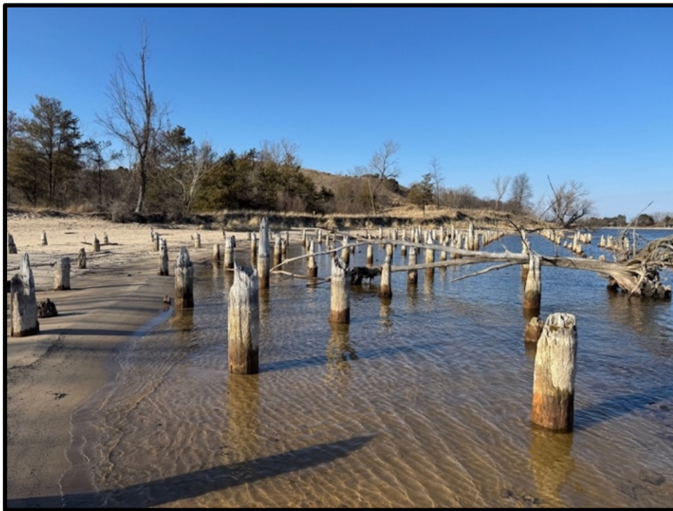
Log pilings from railroad complex of 1858. William Martinus
